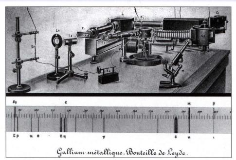
Figure 6. The spectroscope of Boisbaudran, with which he studied gallium, the rare earths, and other elements.<sup>3</sup> His spectrum of gallium appears at the bottom.
